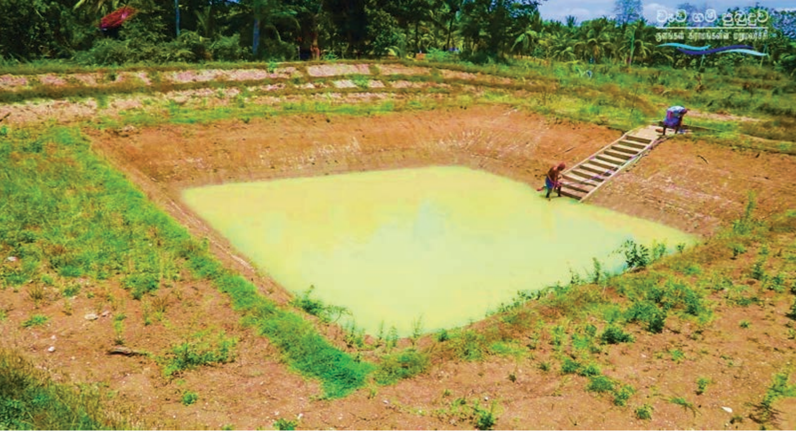
Pathaha, a large runoff water collection tank
