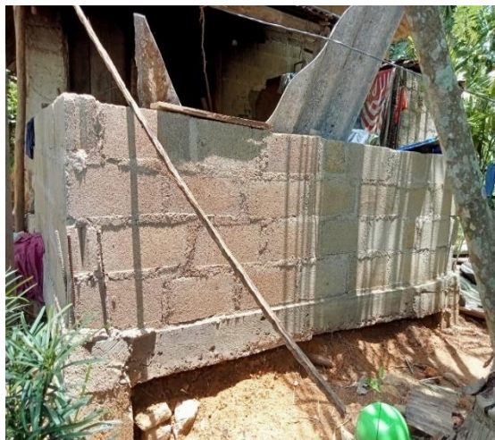
Damaged wall undergoing repair works – Rathnapura District (Photo: SLRCS)
